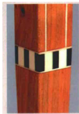
Cuff inlay, which is a band encircling a leg near the floor, is the traditional termination for string inlay.
