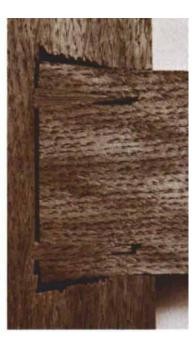
Lay out and cut the joint as you would a standard blind mortise-and-tenon. Then taper the mortise, kerf the tenons and make the wedges following these basic guidelines:
