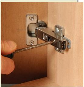
Adjust the door horizontally. There are two screws on the hinge for horizontal adjustment. One moves the door in and out; the other moves it side to side.
