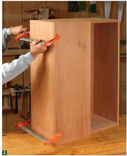
**Clamp the door to the cabinet.** After the plate is clipped in, set the door in place and hold it with two bar clamps. For an inset door, use shims to create even gaps. Leave the second door off for now.
