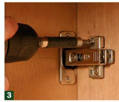
**Attach the plate to the cabinet.** Lean through the opening and drive home the screws.
