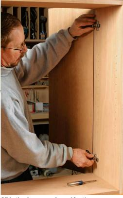
Slide the door up or down. After the screws are loose, it's just a matter of adjusting the door up or down until it's perfect, and then tightening the screws.
