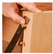
**Peg the joints.** Saw off the waste, and use a sharp block plane to bring them flush.
