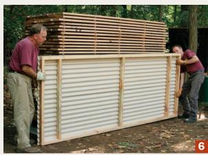
Add a top. A roof made from corrugated plastic over a 2x3 frame (6) helps shield the stack from rain and direct sun. Wrapping the stack in shade cloth keeps out much of the rain, yet allows good ventilation (7).
