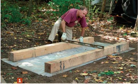
Base of the base. Two 8-ft.-long timbers, which serve as the foundation for the base of the stack, must be parallel, flat, and level. A sheet of plastic under the timbers helps protect the stack from ground moisture and undergrowth.
