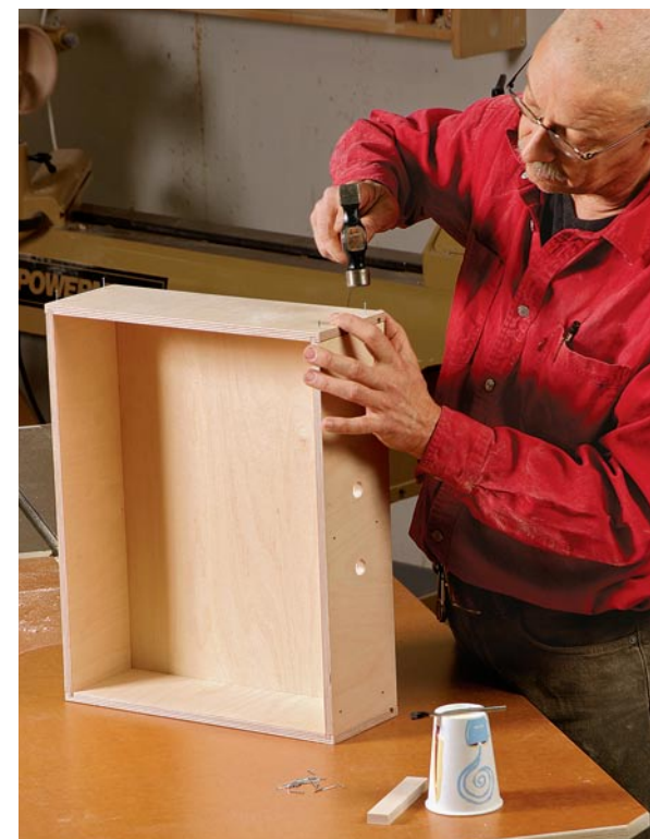
Assembly is easy. Go easy on the glue to avoid squeeze-out. Use brads to hold things snug as the glue dries.
