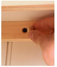
Cover up screw holes. This tea-stained and milk-painted wall cabinet was hung by screwing through an internal hanging rail into the wall. Counterbore the screw holes and insert removable plugs to cover the screw heads.
