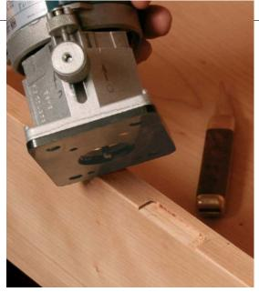
Rout the face frame. Rout close to the layout lines again. and finish with a chisel. Then check the fit on the knob side of the door, or between doors if there are two. Remove the door(s), trim that final edge, and then reinstall them. You should have perfect gaps all around.
