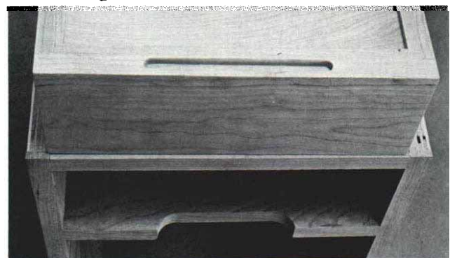
A finger pull that Frid routed in the drawing-table drawer front would have exposed the groove into which the plywood bottom is normally let—a problem Frid solved by gluing a slip to the front, as well as to the sides. The carcass rail, visible at the bottom of the photo, is relieved to give access to the pull.
