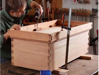
Add the bottom, then the base. With the case upside down, glue and screw the bottom to the case sides. Then set the base in position and screw it to the bottom using the screw blocks.
