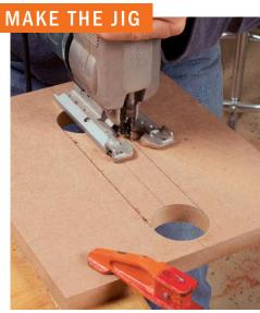
**Cut out the window.** Start by drilling two big holes with a 1<sup>3</sup>4-in.-dia. Forstner bit. Remove material between them with a jigsaw.
