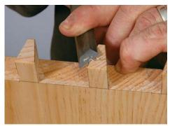
**Tiny chamfers are a big help.** Chamfered edges give the proud dovetails a distinctive look and also make assembly go more smoothly.
