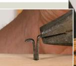
**Clinch the deal.** With the pins linked, push one through the back, the other through the lid. With the lid closed, use pliers to crimp the ends of the lid pin and clinch it with a hammer. Then open the lid and crimp and clinch the mating pin.
