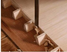
**Chop and pare.** Chop away the waste between the pins with heavy blows, leaving <sup>1</sup>/16 in. or so along the baseline. Follow with paring cuts, starting with the tip of the chisel in the score line. Work from each face of the workpiece toward the middle to avoid blowout.
