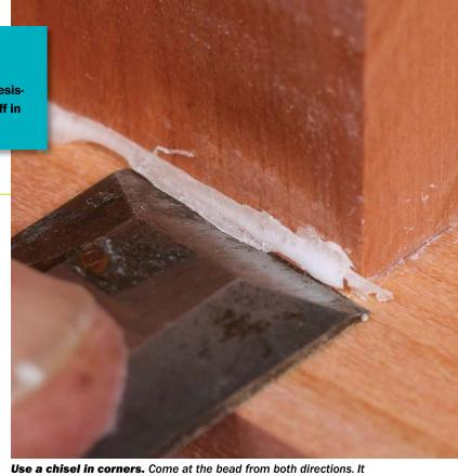
**Use a chisel in corners.** Come at the bead from both directions. It should just fall away. If not, give it a little pull with your fingers.
