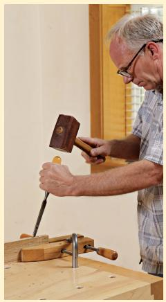
**Chop.** The key to effective mortising is to let the long bevel of the chisel make shearing cuts. Start ½ in. in front of the hole, with the chisel bevel facing away from you. Angle the handle toward you when chopping so the bevel is plumb. Drive the chisel ½ in. or so deep.
