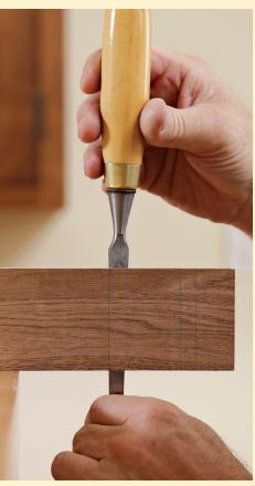
Mortise the other edge and check the ends. Repeat the mortising steps on the other edge. Once you're through on both sides, scrape away any remaining debris until the chisel can extend to the interior pencil lines.
