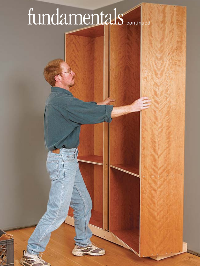
Surface perfection. Using a furniture-grade, cherry plywood for this built-in gives a fine furniture look without the warping and instability of solid wood. Plus, it's less expensive and easier to work with.
