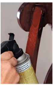
**Apply the ground color, then seal it in.** Wipe on a dye that closely matches the predominant color of the undamaged areas (left). Spray on a coat of shellac to isolate the base color (right).
