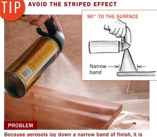
Because aerosols lay down a narrow band of finish, it is more difficult to overlap adjacent strokes, but failure to do so leaves a striped effect on the surface.
