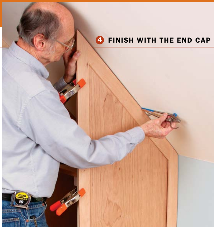
Scribe, fit, and glue it in place. To correct the small gaps on the end cap, Becksvoort runs a compass along the surface of the ceiling (above), transferring the undulations to the frame stock. Then he uses a block plane to shape the frame to that line (left).
