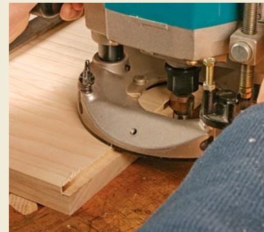
Mark and cut the rabbet. First, mark the rabbet location on the end of the shelf (left), then use a bearing-guided rabbeting bit to cut the rabbet (above).
