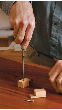
**Add the buttons.** The lip of each button slips into a groove in the apron. It takes just a single screw to secure the button to the underside of the top.
