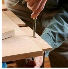
**Elongate the holes.** With the breadboard ends removed, use a marking gauge to scribe a pair of lines tangent to the end holes. A round file or rasp is ideal for elongating the end holes, but stay just inside the lines.
