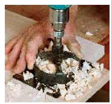
**Keeping square.** The housing helps keep the bit square to the door as the hole is drilled.
