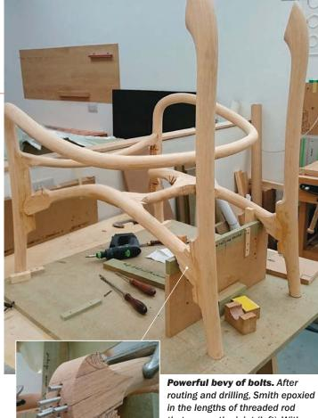
routing and drilling, Smith epoxied in the lengths of threaded rod that secure the joint (left). With the joinery complete and much of the frame shaped (above), Smith finished up with hand tools.
