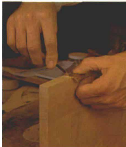
For best fit, hinge mortises must be accurately laid out. Here the author uses a knife to trace the hinge outline to the door stile.
