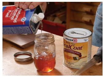
Thin the shellac for easy application. A one-to-one ratio of SealCoat, a dewaxed blond shellac, and denatured alcohol lets you wipe on thin coats that dry quickly.
