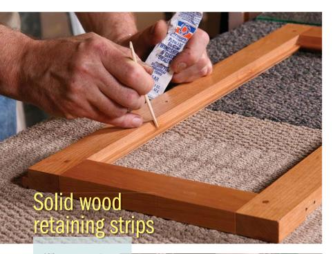
Silicone seats the glass. Whether he's using glazing compound or wood strips to secure the glass, Latta starts by tacking the pane in place with a few spots of silicone glass sealant (above).
