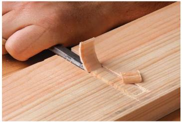
**Rough out the waste.** Use a bench chisel to pare out the waste between the sawcuts, stopping a little short of the bottom. Don't push too hard at the stopped end or you could chip the wood past the stopping point.
