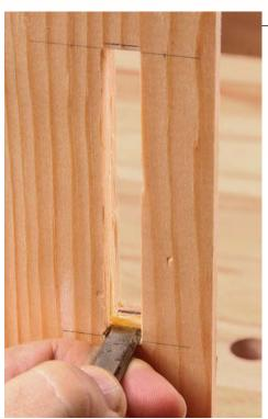
Flare the mortises. Mark both ends of each little taper. One mark goes on the outside face, and the other goes inside the mortise. Connect the marks with chisel cuts.
