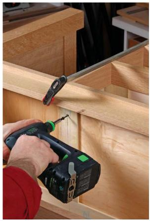
**No joinery means easy addition.** The drawer-divider assembly sits on the case bottom. Lower it into place (left) and then clamp it there. Lay the case on its back, and attach the divider assembly with screws driven up through the case bottom (above). Two screws on each side are enough.
