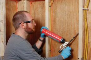
No matter where you live, seal and insulate. Spray foam along the studs (top), and caulk between the floor joints (right) minimizes air movement between the inside and outside, while insulation (below) helps keep the shop cool in the summer and warm in the winter.
