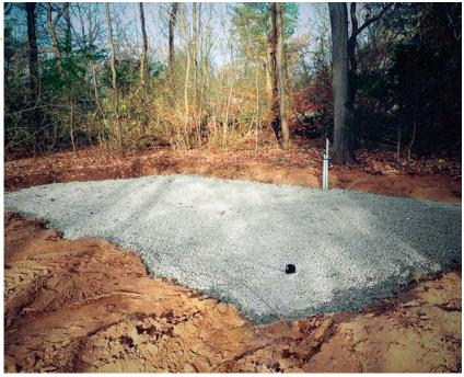
**Firm, level foundation.** The crushed stone used to support the shed is easy to level, but the ground beneath needs to be level, firm, and flat, too. That's where the hard labor is.
