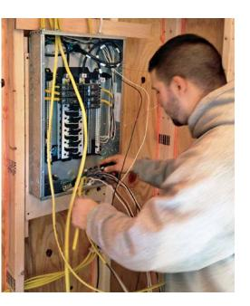
run circuits for lighting and outlets. I had worked out where I was going to put all of my tools beforehand, so I gave the electrician a map identifying where I wanted the outlets and boxes for the lights.
