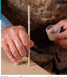
Add epoxy. Fortune uses a small dowel to spread it over the hole's wall.
