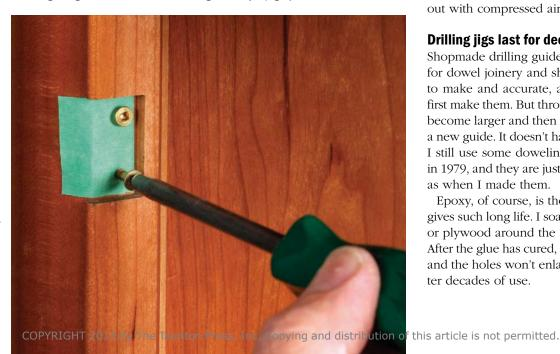
are infused with hardened glue. I've found that the best way is to cut the threads with a tap. If you form the threads by driving the screw into a pilot hole, the screw simply pushes the fibers into the shape of the threads. This burnishes the wood, making it less absorbent. If you cut the threads with a tap, more epoxy can soak in.
