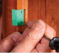
Cover with tape. This prevents the wet epoxy from pouring out of the holes (left). A small hole created by an awl is enough to get the screw started through the tape (right).
