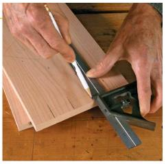
**Transference.** Use a square to transfer the center marks of the pin sockets to the end of the board.
