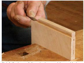
Notch the top end. Use a backsaw and then a chisel (above) to cut away 3/4 in. or so at the top end of the dovetail, creating an angled surface that mates with the slightly curved inside face of the drawer front (right).
