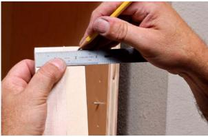
but leave the stiles overwide, unattached, and with the biscuit slots already cut. That way I can scribe the stiles to the wall and cut them while they're loose, which is easier. Then I use the friction from the wall, rails, and biscuits to help hold the stiles in place while the glue sets.
