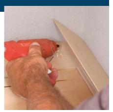
**Glue them together.** Zall uses hot-melt glue to attach the template sides to the back piece. Before removing the template, mark where it meets the cabinet's front edge.
