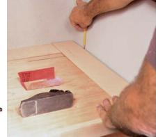
**Scribe each piece.** Butt the edges of the MDF pieces against the wall and use a pencil as a scribe. Then trim the edges down to the line using a block plane.
