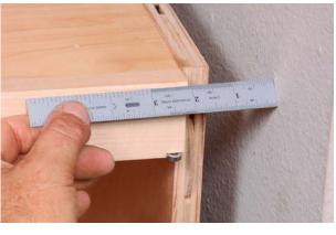
Transfer the distance. Run a strip of masking tape along the edge of the stile to help mark and trim the edge without marring the piece. For now, just transfer that top distance.
