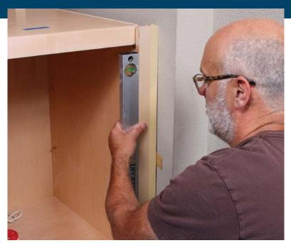
**Keep stiles plumb.** Lay the stile on top of the rail and butt the rabbeted edge tightly against the wall. Check it with a level and shim if needed.
