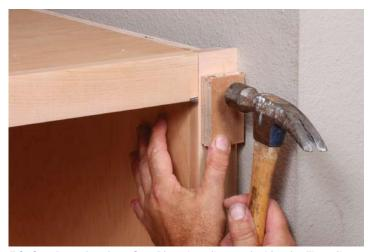
**Friction does the clamping.** Pivot the stile onto its biscuits. The rails and the wall will keep it wedged in place while the glue sets, but give it a couple of taps first to get it flush.
