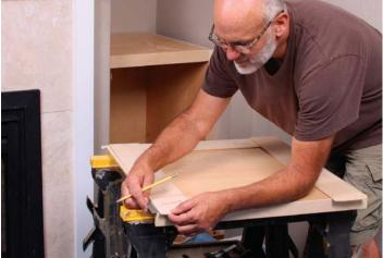
Line it up. Use the marks at the front to align the template, adding an extra 1¼ in. to account for the overhanging top, and trace the template. Use a fine-tooth handsaw to cut through the maple cleat in the front but remove the rest of the waste with a jigsaw and trim the top to fit with a block plane.
