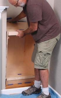
**Lock it in place.** Install the cabinet equidistant from both side walls. Push it against the back wall again, shim any gaps at the back edge, and screw through the top of the back panel into a wall stud.
