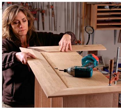
Fit and install the crown. With all the miters cut, Hiller positions the front piece of crown and secures it with countersunk screws. Then she puts glue on the miters, putting the return pieces in place and clamping the corners with Ulmia miter clamps before securing the return pieces with screws.
