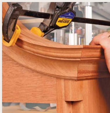
A fussy fit. Sometimes the miter joint fits right the first time. If not, you may need to trim the cuts or modify the profile until the corner comes together.
