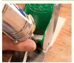
**Seal the mouth.** First, put painter's caulk into the mouth to keep water and abrasive grit from getting under the riveted sole, where it will be hard to remove.
