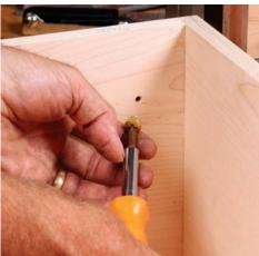
Install the stop. Transfer the mark from the top of the slide to mark the drawer side for drilling (left). Drill with a 3/16-in. Fuller taper bit, cut the threads with your standard tapered tap, and then insert the stop (right) from inside the drawer while the drawer is resting on the slides.
