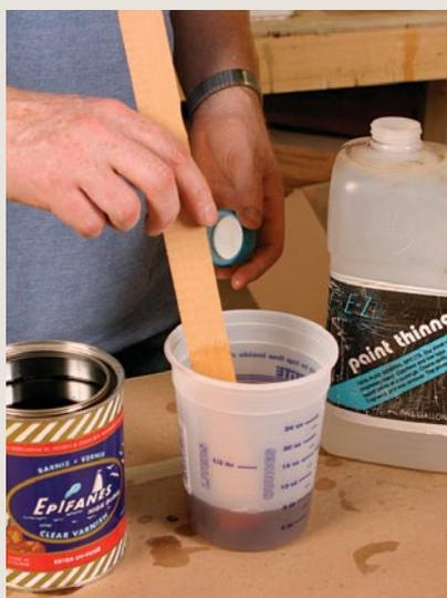
**Thin the varnish.** To promote better absorption, thin the first three coats of varnish with mineral spirits. When applying, take care to cover all the surfaces.
