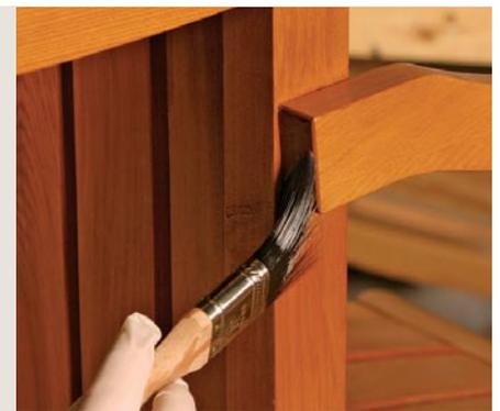
**Apply the primer.** Once the two-part epoxy is combined, you have about 20 minutes to apply it generously to the surface, letting it saturate the wood. Pay attention to the end grain as this is where weather damage is most likely. Re-coat these areas as the epoxy is absorbed into the wood.
