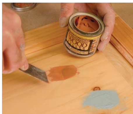
A smooth surface. Large holes are best filled with an auto-body filler that must be mixed with a hardener (far left). Fast-drying wood filler is ideal for medium-size holes (near left).
