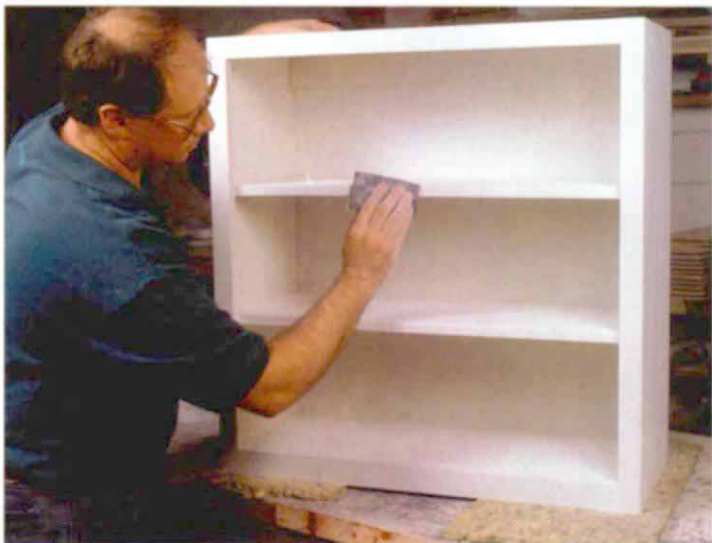
Sprayed finishes are only as good as the surface below. The author primed this bookcase and now sands it with 220-grit paper in preparation for spraying on a tinted waterborne lacquer topcoat.
