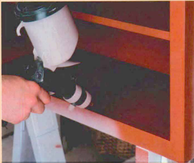
4 Finish the face frame. Begin with the inside edges, and then move to the front of the case.
