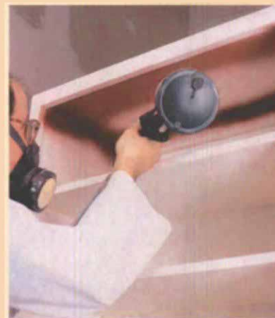
1 Spray overhead corners, and, then fill in the inside top.
