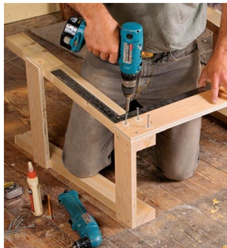
Glue and screw parts together. Finn sinks only one of the four screws, then adds the others once he squares the long stretchers to the leg assembly.
