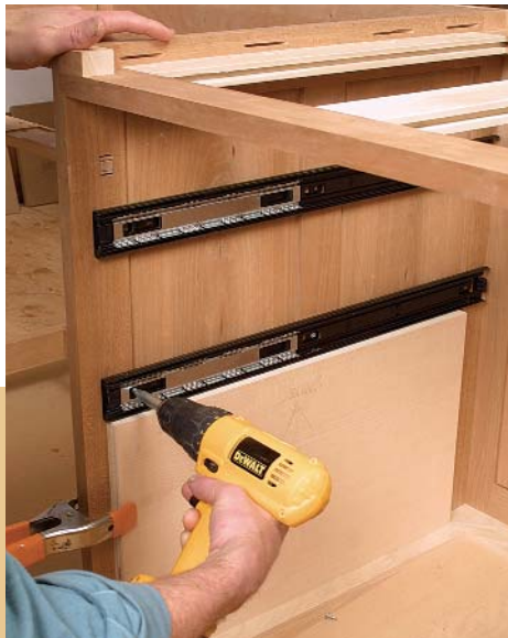
Install the drawer-slide hardware. Rest a piece of plywood or MDF inside the cabinet to locate each pair of slides. Start with the highest slides and then trim the plywood to locate each set below.
