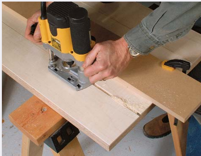
Rout the joint. To clean up any gaps, a router and edge guide are used to cut a shallow groove centered on the long joint.
