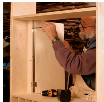
Attach the inner doors. Stretching from the top of the gallery to the bottom of the upper shelf, each inner door is hung from a post screwed to the cabinet.
