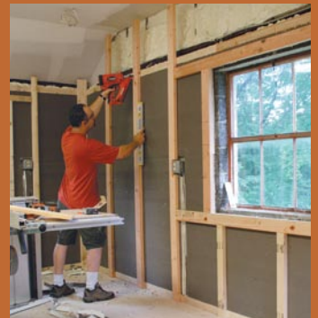
4. Insulate the walls
