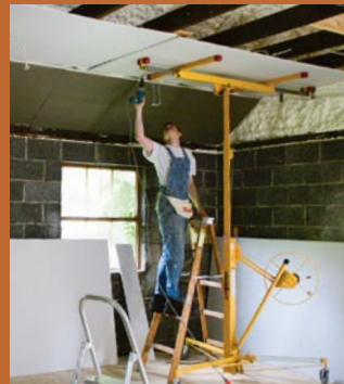
3. Finish the ceiling
