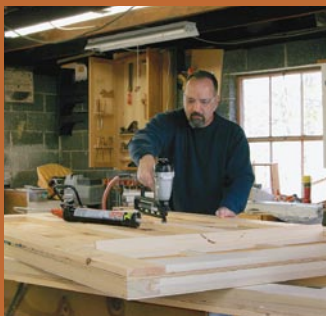
1. Install new doors
