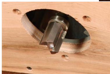
Cut away high spots. A plywood sled holds the router as it's moved from side to side. A 1-in. straight bit (inset) quickly removes the waste. When one side is relatively flat, turn the slab over and flatten the other.
