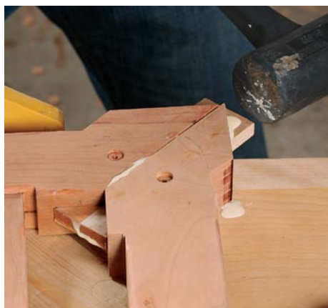
Knock in the spline. With so much glue surface, it takes a bit of force to get it all the way in. Keep your mallet blows straight to avoid breaking off the spline.
