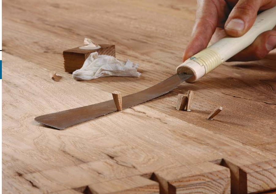
Plug holes with scrap. Chisel random-shaped pegs from offcuts and glue them into nail holes or worm holes (left). Then trim them flush (above).
