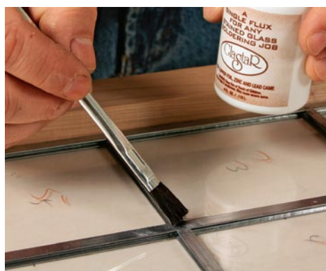
Flux first. Flux cleans the joint before soldering. It also helps the solder to flow more easily when it's melted, making a better-looking joint.
