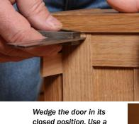
Wedge the door in its closed position. Use a square to determine the proper inset and slip some shims between the case and door to hold it in place for drilling. Use a stop block on the drill to prevent drilling too deep.
